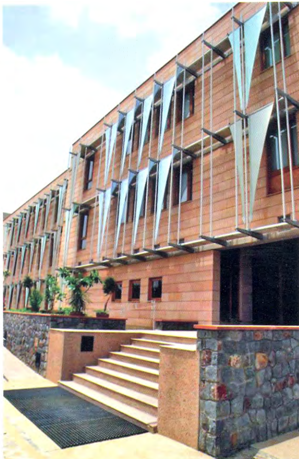
Natural light is modulated through fixed blinds and based on the positioning of the building.
